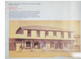
In 1923, an extra storey was built and added using the same Girzi stones to match the stonemasonry of the building.
