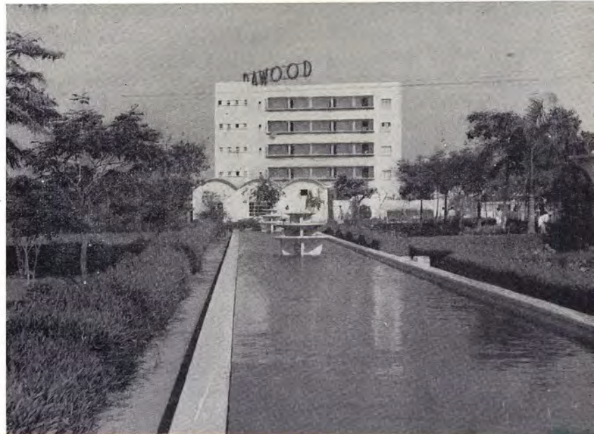
A view of the five-storied hostel
